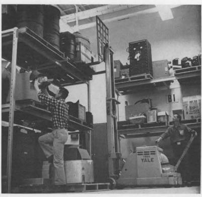
MATERIAL STORAGE in Bldg. 870 is achieved with maximum efficiency utilizing these space saving racks. Racks are movable and allow flexible space arrangement. At left Flaviano Saavedra places material on the rack while Willard Randall uses fork lift to remove items from top shelf. Material is awaiting processing.
